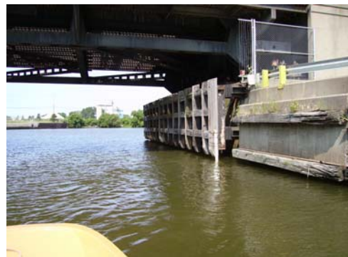
Figure 2.3 Site 2, Ohio St. Bridge.
