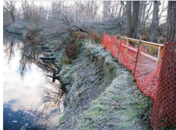
Photo 4.1-5 Stiglmeier Park bank failure, sediment loading, and loss of riparian habitat
