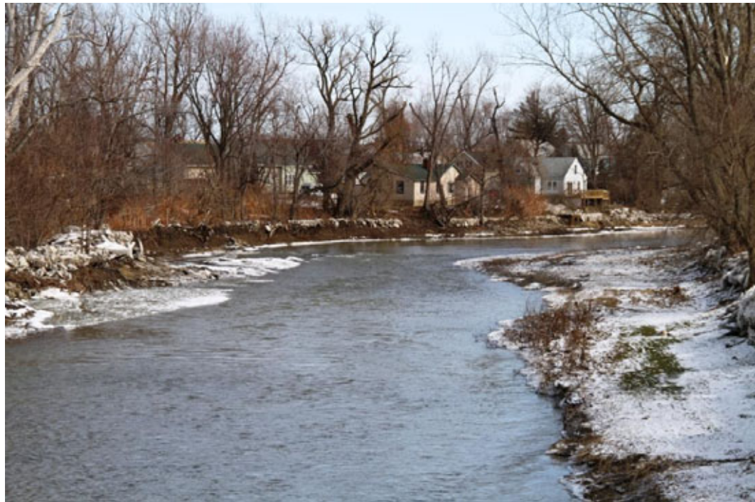
Photo 4.3-1 Cazenovia Park site continual bank failure, observed on February 21, 2011
