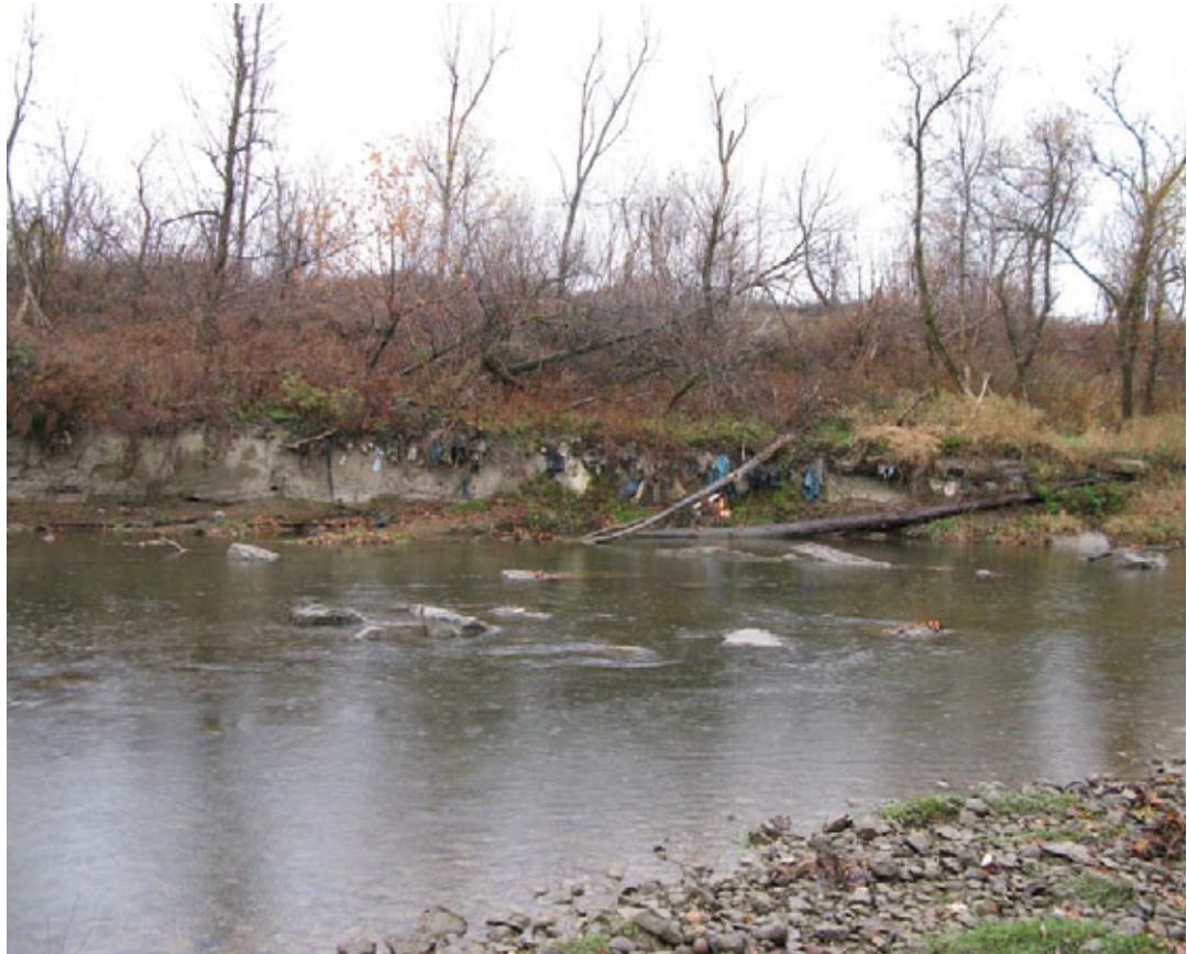
Photo 5.3-3 Cayuga Creek stream bank failure and sediment loading
