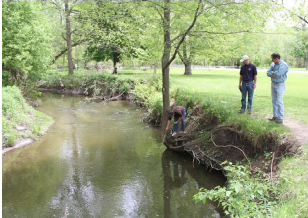
Photo 5.2-2 Data collection of hydraulic shear stress, stream bank stability and fishery baseline conditions for monitoring
